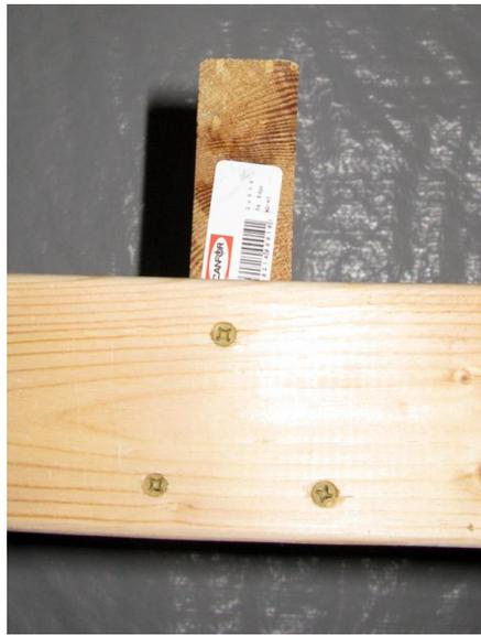
Side View – (3) screws per side, (2) two in the 2”x4” and (1) one in the 2”x6”
